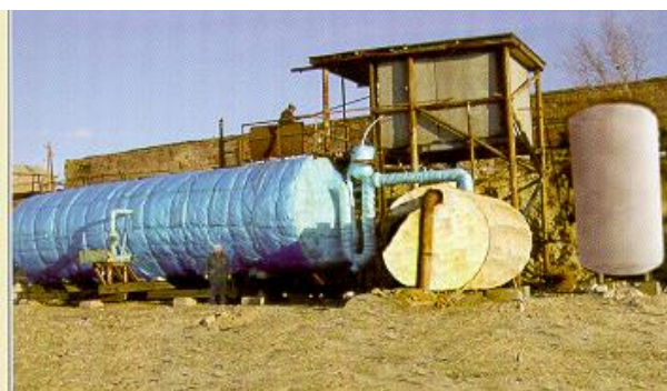
Figure 14. Biogas plant in Bartsrashen, Armenia (bioreactor 52m 2 )
