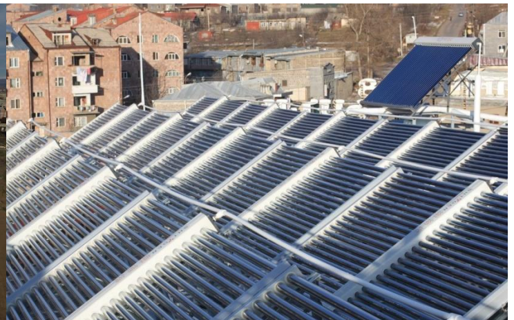
Figure 10. Solar water heaters at the roof of Hotel Diana in t. Goris installed by Shtigen Co.
