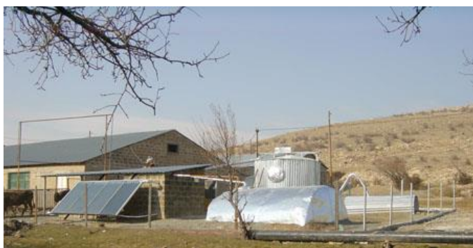
Figure 15. Solar integrated 25m 3 digester based bio-gas pilot project at farms in Arzni village
