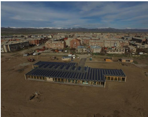
Figure 9. 95kWp PV station in Armenia was installed in Gyumri in 2014 by Caritas Armenia NGO
